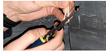
The wires are then inserted into the terminal block and secured with a Flathead screwdriver. Wrap the terminal block, wires, and insulation with fibreglass tape to prevent the wires from coming in contact with the firebox
