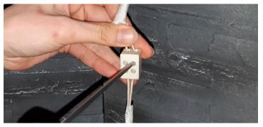
Insert the light back into the firebox ceiling as shown below, note the securing tab on the wired side of the light.
