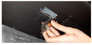
2 Cut the 2 wires from the dead or damaged light, then using a stripper, remove 1/4" of insulation from the wires and twist.
