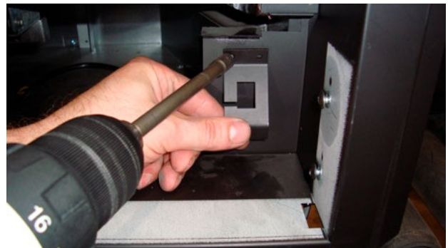
Figure 6 Attach switch bracket to front of fireplace
