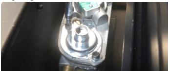
10. The pilot size can be adjusted using a flathead screwdriver to adjust "pilADJ" screw shown
