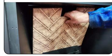
If necessary, remove the baffle at the top of the firebox to ease the install of the liners. Baffle must be reinstalled once liners are in place.
