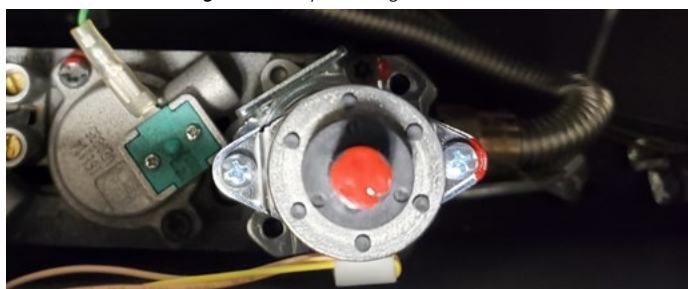
Figure 13.eee LP pressure regulator on a Full Load
