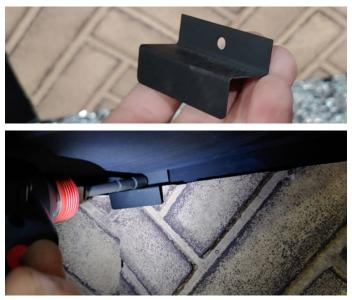
Figure 20.b Secure with the bracket using screw
