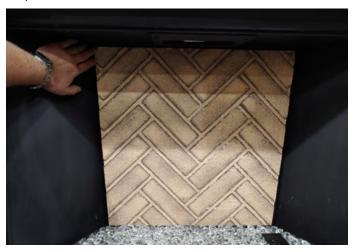
Figure 20.b hold in place or secure using masking tape
