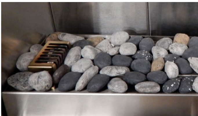
Figure 68 Ensure the stones DO NOT cover the pilot.
