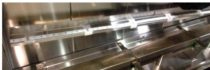
Figure 43 Adding LED air baffle
