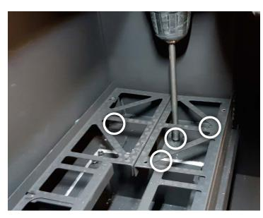
Remove the firebox pan being secured with twenty (20) #8 tek screws. The pan can now be pulled forward and gently rested on the front lip of the fireplace frame.
