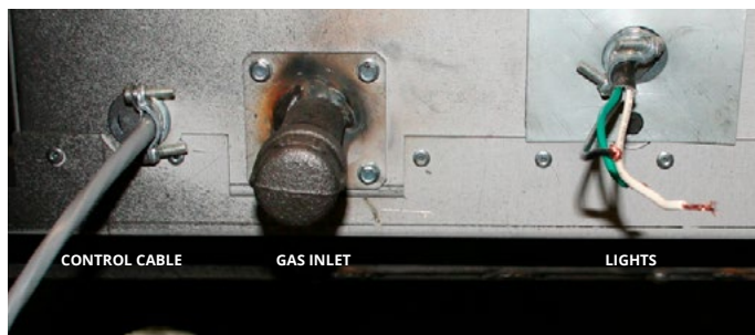
Figure 9.b.b Identifying the Gas Inlet
