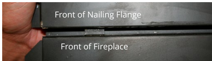
Figure 4.e Insert folded tabs into slots above the front of the fireplace
