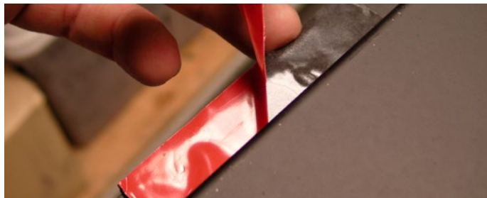
Figure 5.12b Peeling self-adhesive tape
