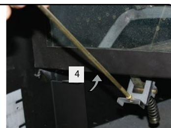
Figure 23.g Lift the door up and out of the fireplace frame
