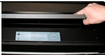
Figure 4.c Note placement of rating plate
