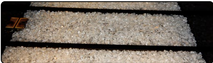
Figure 7.b Completed fireglass installation
