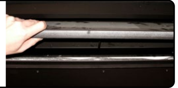
Figure 4.f Exposing controls under control panel
