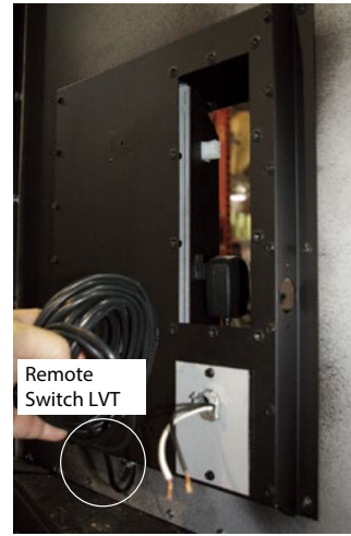
Figure 12f. Installing the Remote LVT Switch.
