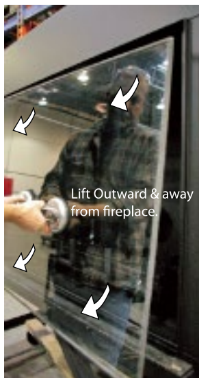
Figure 17. (Lift the door upward)
