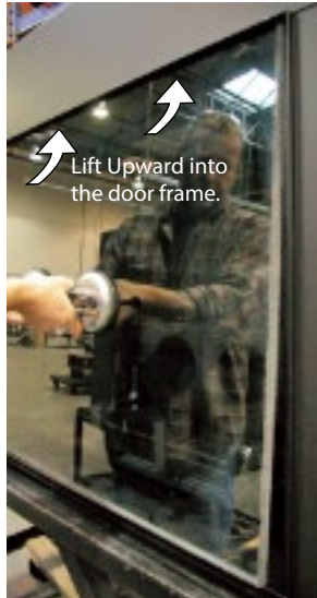
Figure 17. (Lift the door upward)
