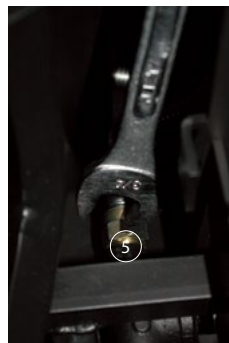
Figure 20d. (Loosening Gas fitting on burner).
