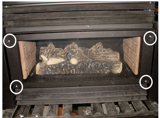
Figure 11b. Removing the screws.
