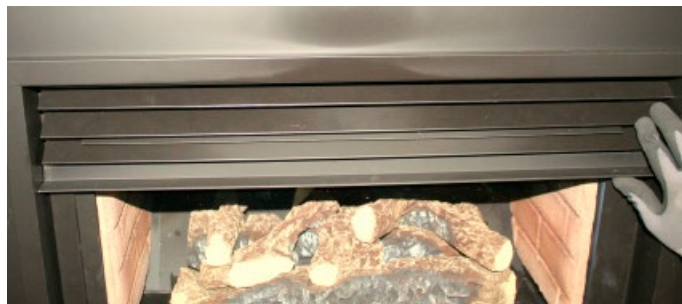
Figure 9c. Completed installation of Upper louvres.
