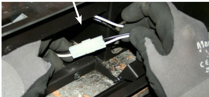
Figure 10b. Connect Fan Speed Control wires.
