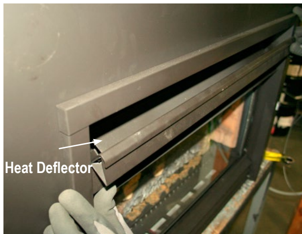
Figure 9b. Installing the upper louvres.
