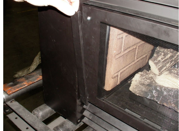
Figure 11a. Removing the screw covers.
