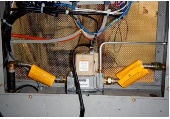
Figure 131. Valve assembly installed.
