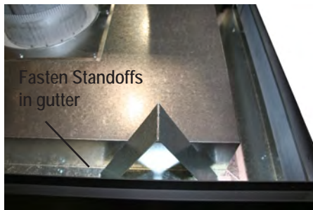
Figure 6. Installing the H*38PR* standoffs.
