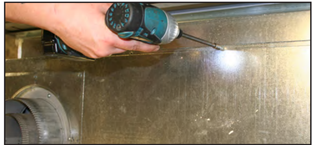
Figure 7. Remove screws from top of the unit
